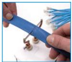
When the knife is hot, slide the sleeving over the cutting blade. Practice on a piece of scrap to get a feel for the procedure. Always cut in a well ventilated area and avoid inhaling the fumes. Both the blade and the cut ends will be **HOT.** Be careful.
